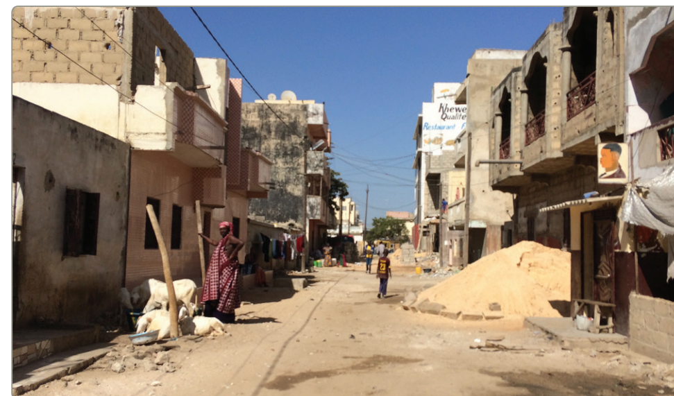
Self-built Neighborhood, city of Pikine in the periphery of Dakar (Source: A. Deboulet)
