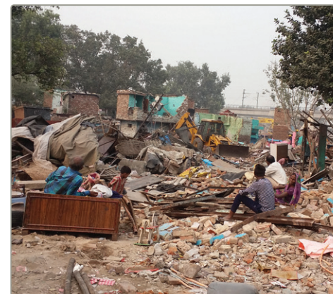
Demolition being carried out in the Kathpuli Colony neighborhood (2700 households) in Delhi (Source: Shankare Gowda, 2017)
